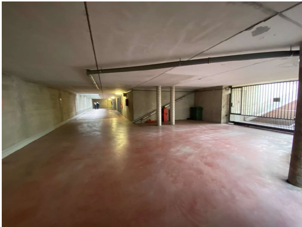
Vista corsello box piano S1
