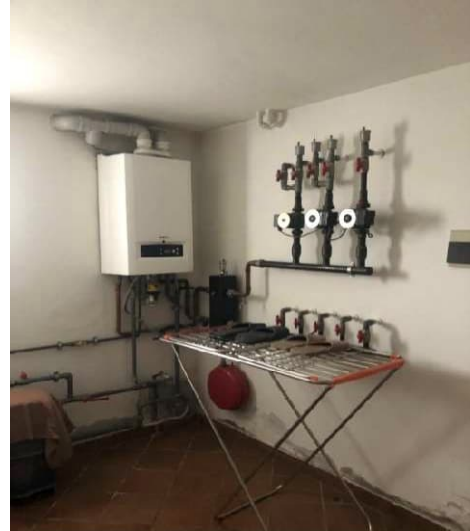
Vista locale C.T.
