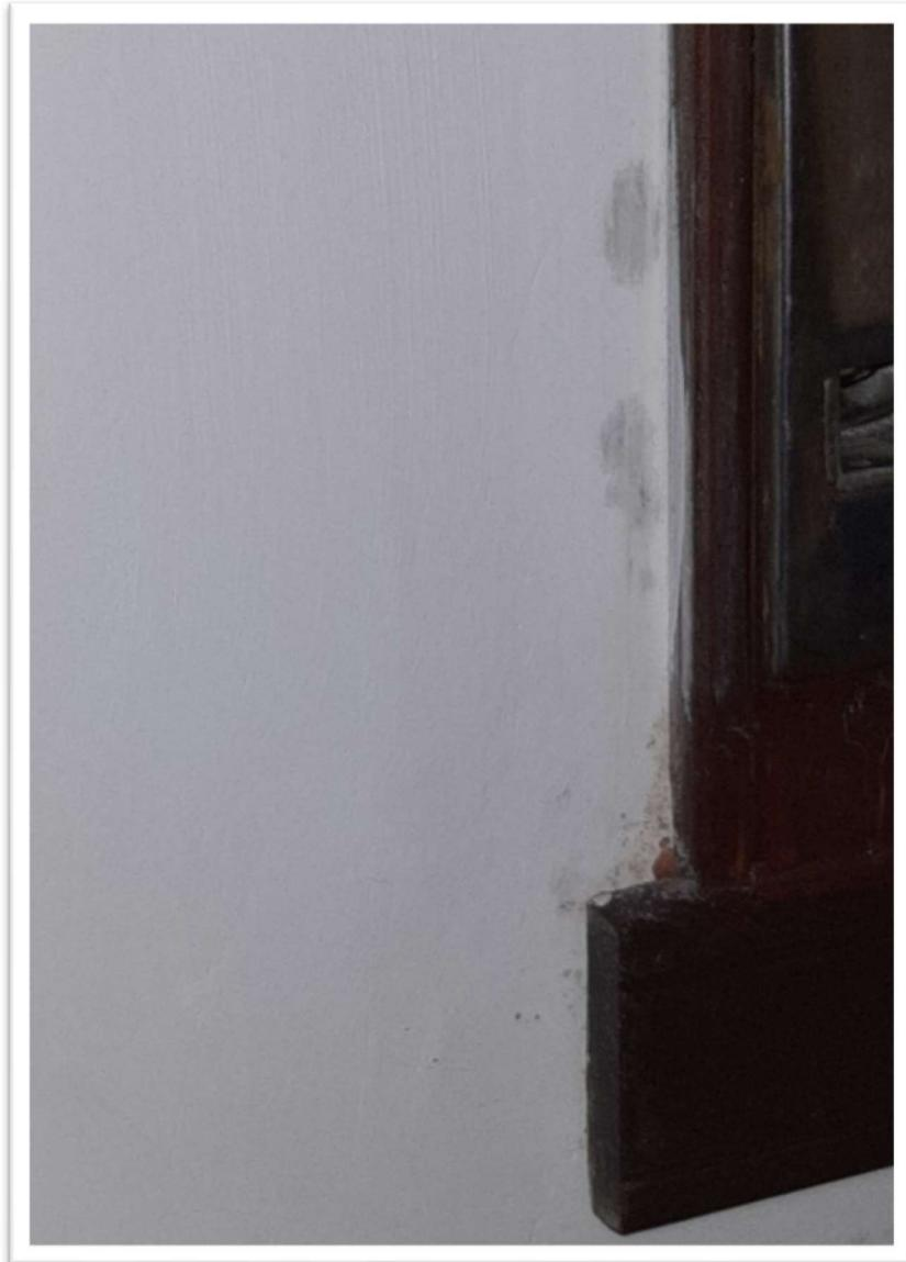
**FOTO 17: PARTICOLARE UMIDITA' TRA INFISSO E PARETE CAMERA SINGOLA**
