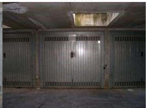
Vista serranda box
