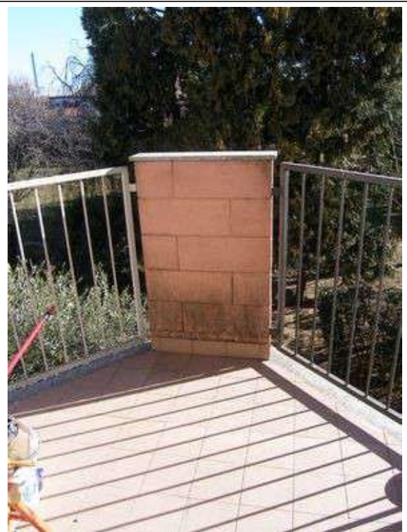
Vista balcone piano 1
