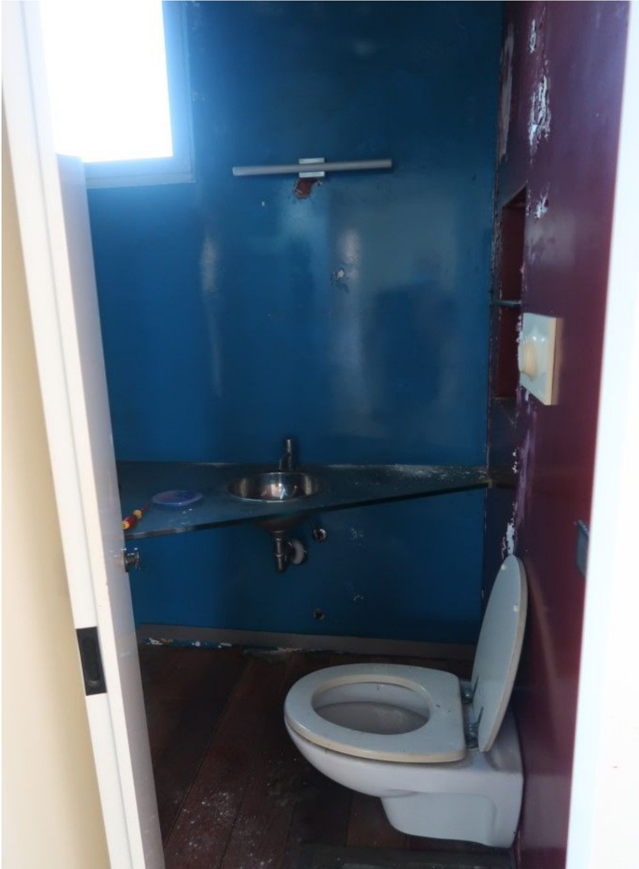
BAGNO PIANO TERRA
