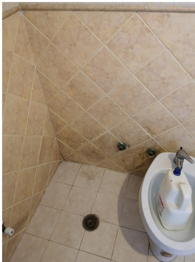
15 - bagno piano terra
