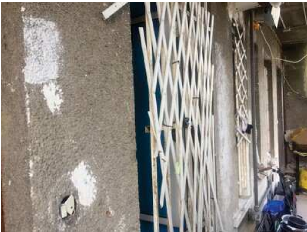
Finiture P3 – Grate antieffrazione
