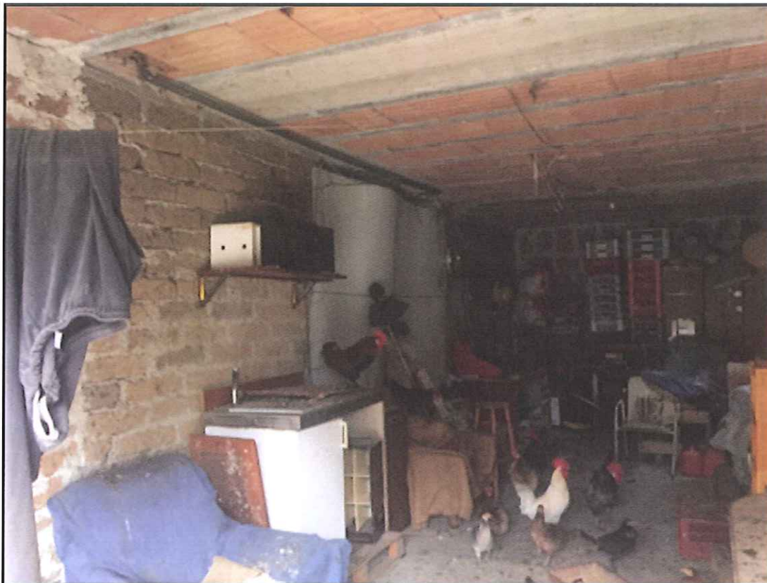
Figura 51: garage al piano S1
