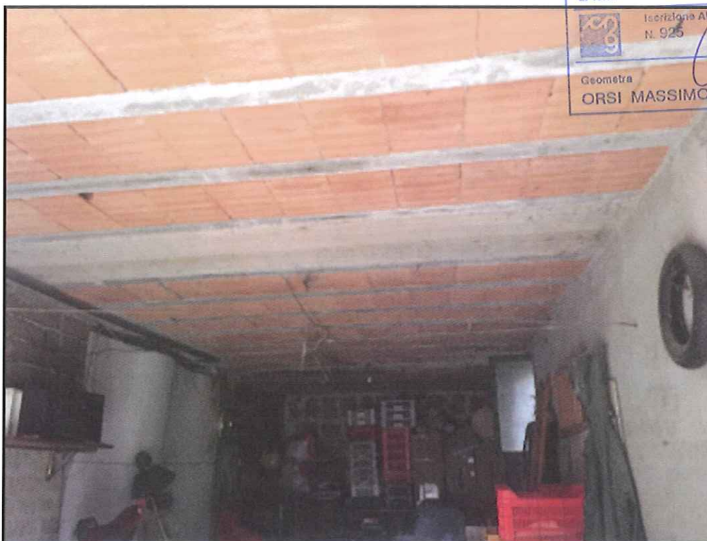
Figura 52: garage al piano S1
