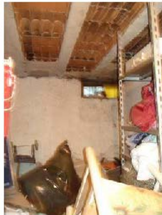
locale piano S-1
