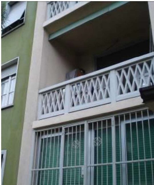
Vista ext/ int veranda
