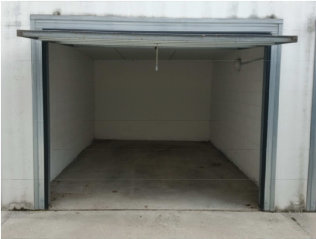
Vista interna garage
