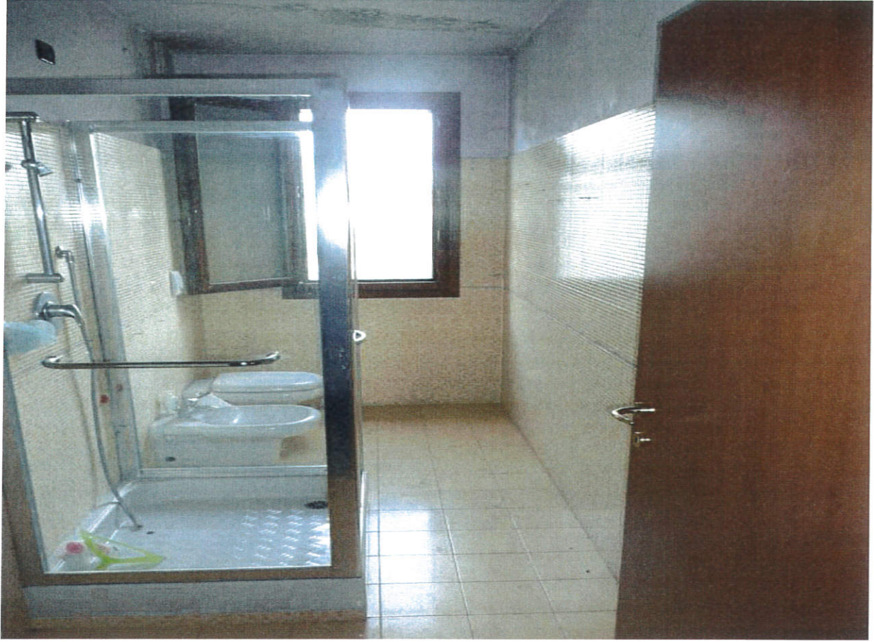
BAGNO PIANO TERRA
