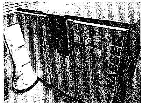
Compressore AS 36 KAESER.
