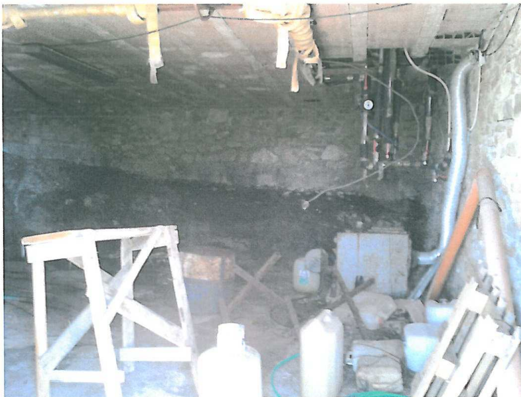
Piano Seminterrato – Cantina
