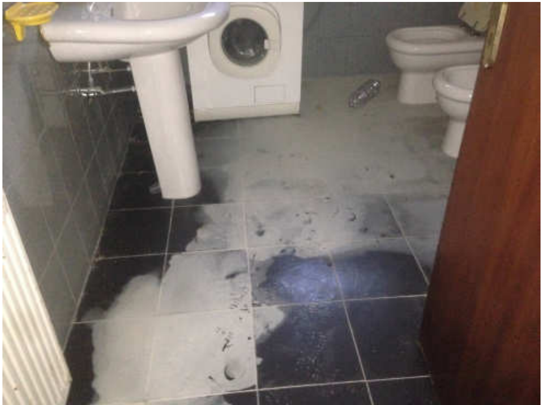
bagno piano seminterrato
