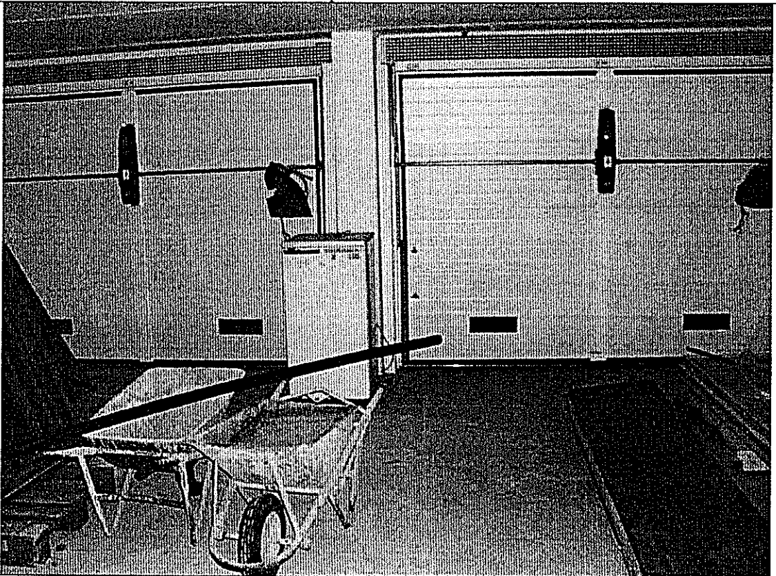
vista interna garage
