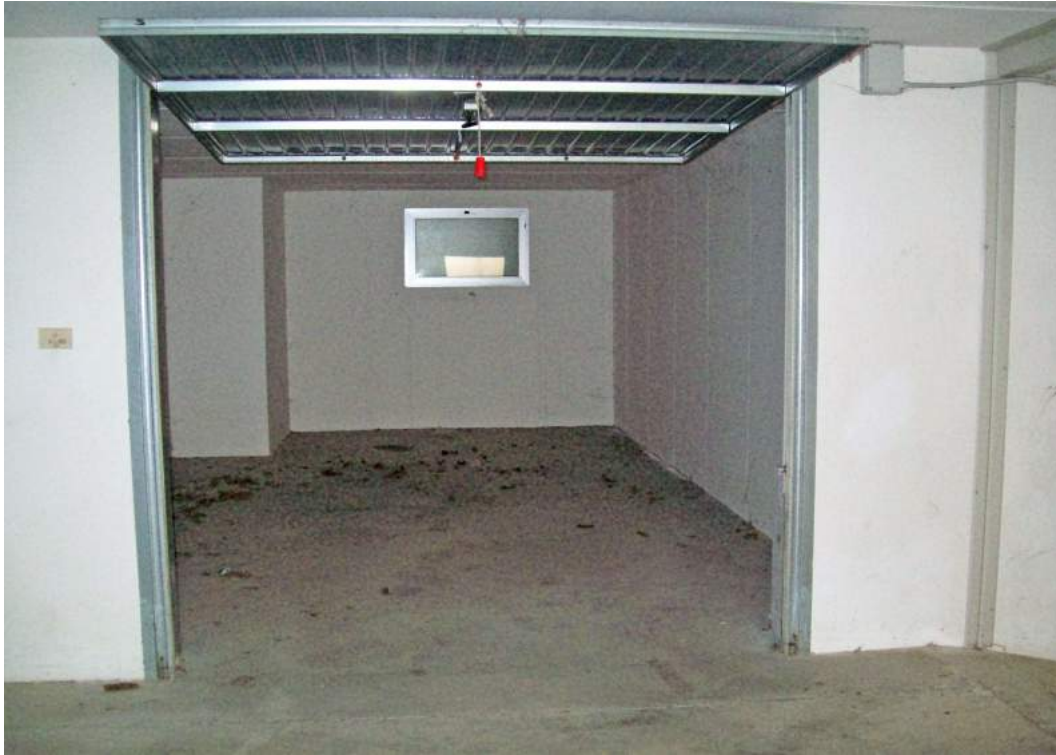
Foto 43a.11: garage piano interrato
