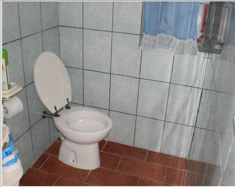
Bagno piano terra
