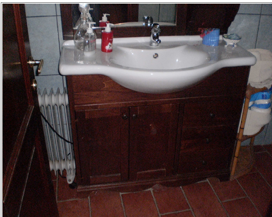
Bagno piano terra
