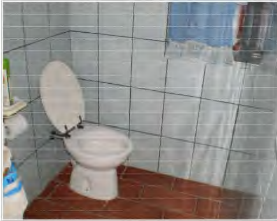
Bagno piano terra
