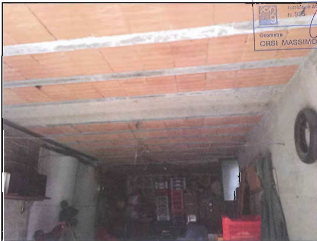
Figura 52: garage al piano S1
