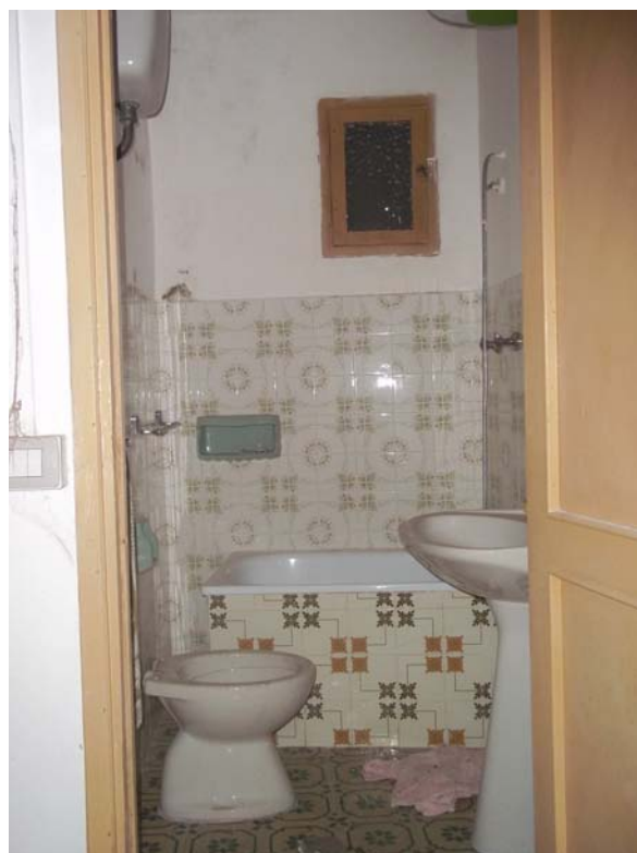
5 – P.Ila 125/2 – Bagno Piano Terra
